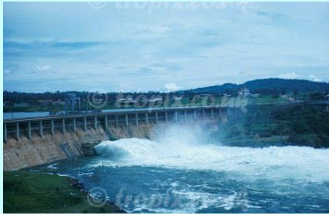
Owen Falls hydroelectric dam, floodgates open, white water rushing; HEP. Nalubaale Power Station, Jinja, Uganda.
