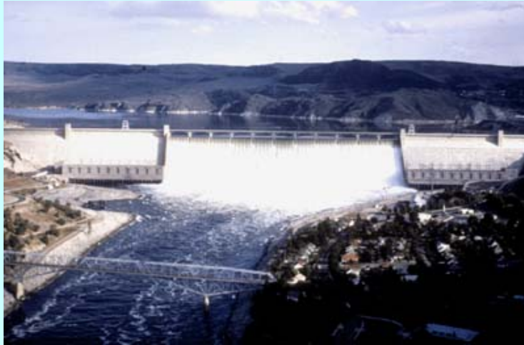
Grand Coulee Dam, Columbia River
