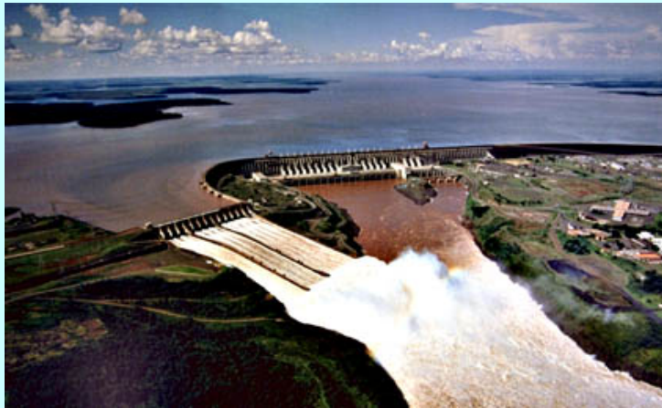
Spillway with rushing water and mist, electricity pylon; hydro power, alternative energy. Itaipu HEP Dam, Brazil.
